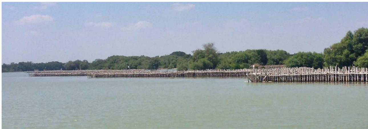
**Building with Nature on the northern coastline of Java uses Hybrid engineering to rehabilitate mangroves. Local materials have been used in its construction, which enables the mangroves to trap sediment and drastically slow down erosion.**
