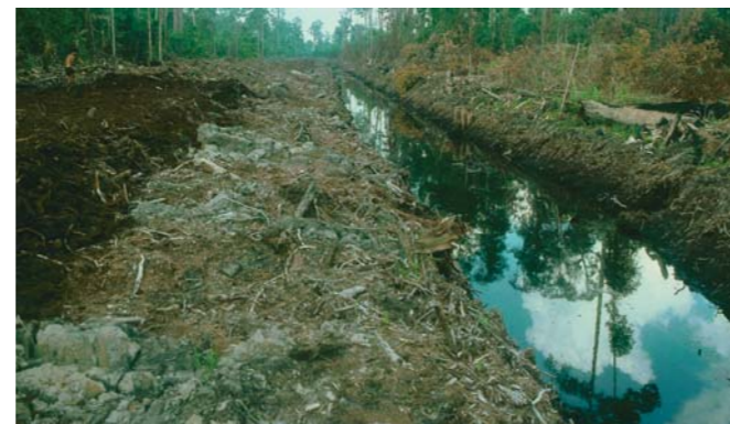
Draining peat forest for plantation development, Riau. (Photo by Christian Cossalter)
